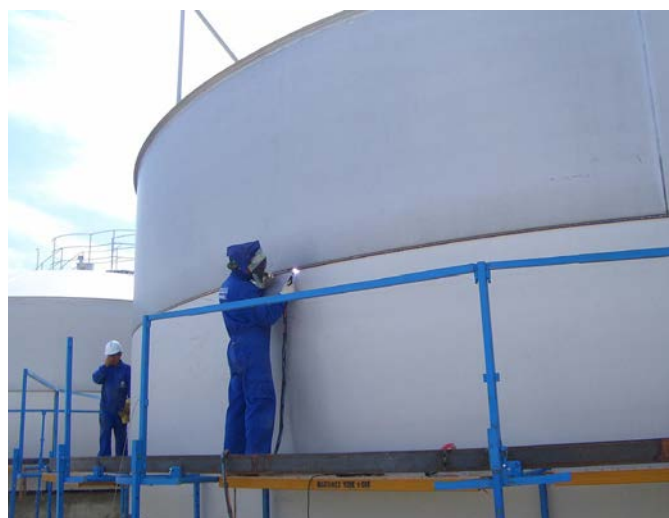
Welding on-site of stainless steel tanks – a typical application of Böhler Welding rutile all-position flux-cored wires. Tanks are in UNS S32101 and welded with Avesta FCW LDX 2101-PW (E2307T1-4/1).
